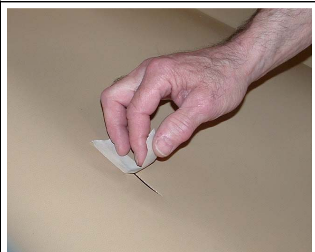
Apply masking tape on the backside of tear.
