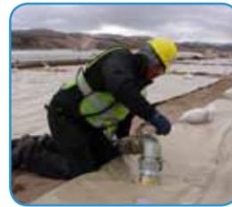
Personnel can now ready the tanks for filling by installing fill/drain valves to isolate individual tanks in the farm. Specialized arctic vents prevent overfilling.
