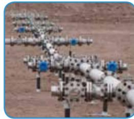
SEI Industries designed a customized fuel system that could face a number of challenges and in just three weeks, it was deployed and filled. The entire system was transported in 20-foot ISO containers. Here, the manifolds system is complete and is waiting to be connected to tanks.
