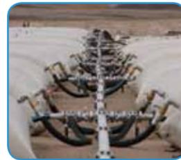
Using an SEI-engineered system, the tanks are filled with fuel through an innovative network of manifolds and pumps. Tanks can be isolated into groups of four or filled individually, if required.
