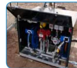
The addition of more SEI-engineered equipment allows for easy fuel handling on-shore. The system's light duty vehicle refueling pumps allows operators to fuel vehicles just like any service station.
