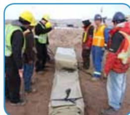
Using 6-8 personnel, unfolding an Arctic King™ tank can be accomplished quickly and easily. Very little training is required, especially once the team experiences the set-up of the first tank. With a team leader in charge, straps are removed and the Arctic King™ tank is soon deployed into its new location.
