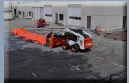
3. Position bobcat for rolling and secure roll bars.
